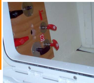
2: Inert gas projection lever
